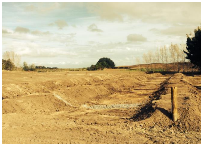
Figure 1: Humps and Hollows for a new planting.
